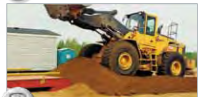
3 Backfill to bulkheads and finish ramps.
